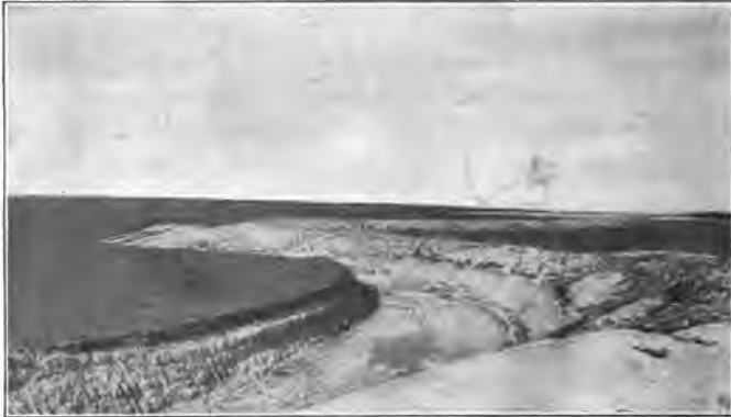
Fig. 68. Riverside Canal in Colorado before the water was turned in for the first time. This canal where shown is 18 feet wide at the bottom.
