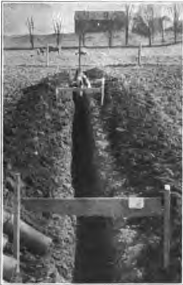
Fig. 57. The target method of grading the ditches.
