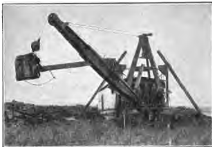
Fig. 66. A floating dredge for digging open ditches.
