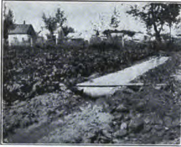
Fig. 72. A canvas dam in use. (Farmer's Bul. 392, U. S. Dept. of Agr.)
