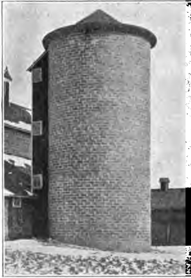
Fig. 296. The Iowa silo made of hollow vitrified clay building blocks or tile.
