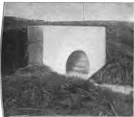
Fig. 63. A good outlet protection for a tile drain. It is desirable, however, that grating or bars be placed across the outlet to keep out small animals.
