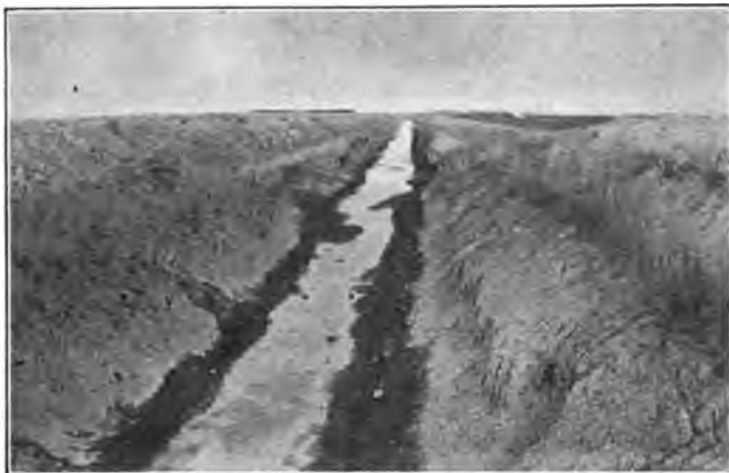
Fig. 43. An open drain.
