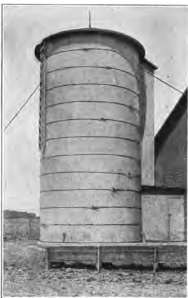
FIG. 294. A good stave silo well anchored.
