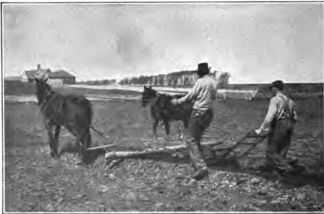
Fig. 61. Filling the ditch with a plow.
