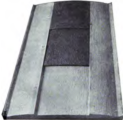
Fig. 83. Model of a gravel road illustrating the trench method of construction. A shows prepared sub-grade; B, first course of gravel; C, upper course of gravel. (Bul. 36, Office of Public Roads, U. S. Dept. of Agr.)
