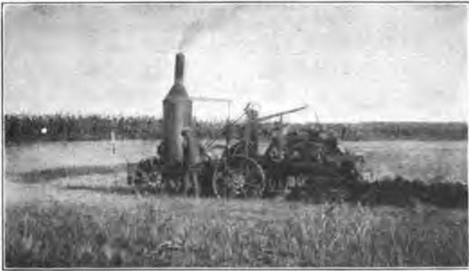
Fig. 54. A tile ditching machine at work.
