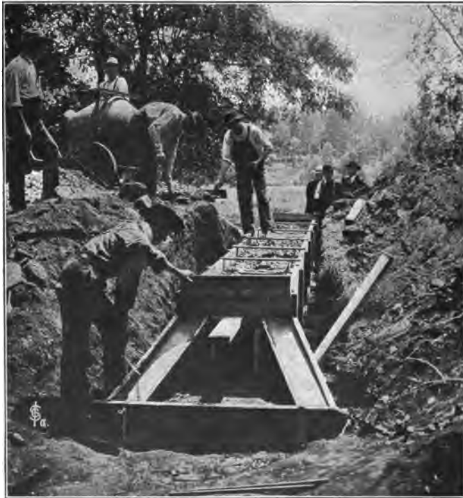
Fig. 95. Making a concrete culvert.
