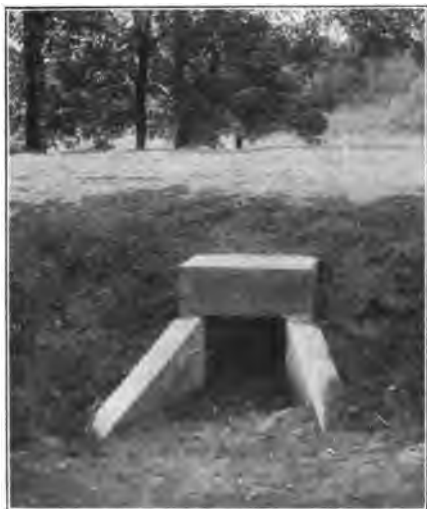
Fig. 97. Concrete culvert after the plan of Fig. 88.
