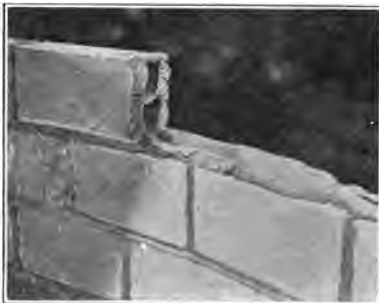
FIG. 297. The wall of the Iowa silo.
