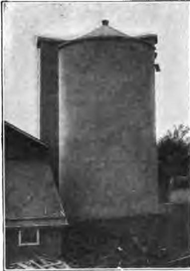
Fig. 295. A monolithic silo with concrete roof.
