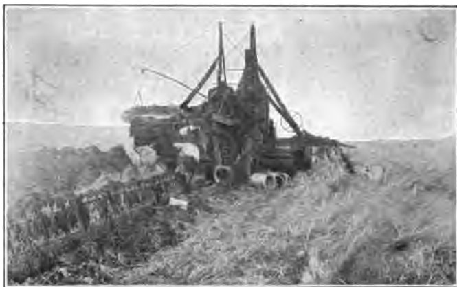
Fig. 55. A large tile ditching machine at work.
