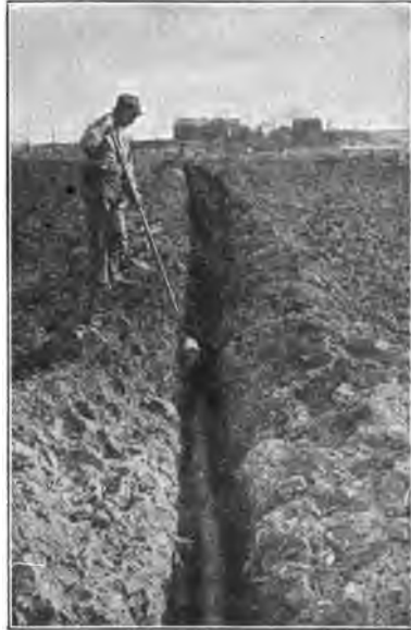
Fig. 59. Laying tile with the tile hook.
