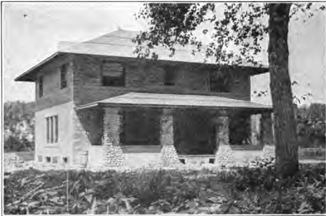
Fig. 293. A concrete block house representing a good type for the farm.
