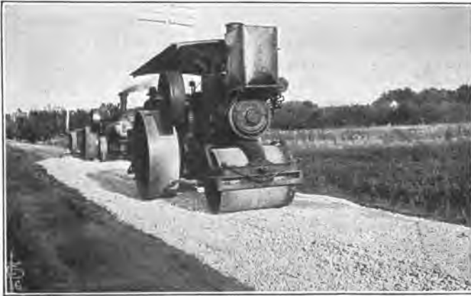
Fig. 84. Rolling the first course of stone.
