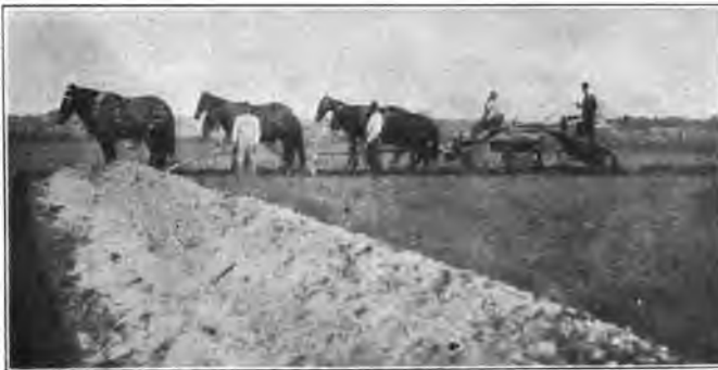
Fig. 62. Filling the ditch with a road grader.
